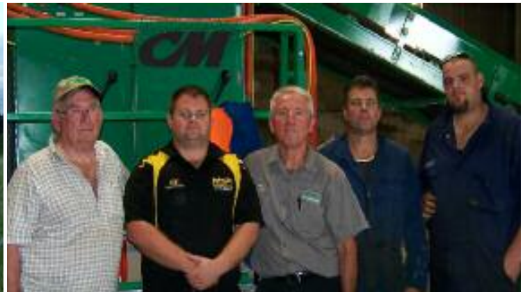
From left; Ray Austin, and Jamie from RBE a local engineering firm along with Ziggy Kotlarczyk, CM and two support staff on site at Tyre Disposal during installation
